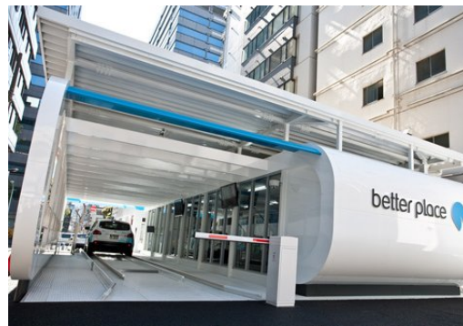
Figure 7.2: A 'Better Place' switch station. [121]
